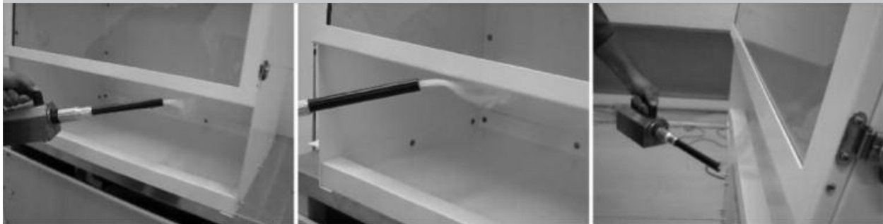
FIGURE 30. AIRFLOW SMOKE TEST – EXTERNAL PERIMETER
