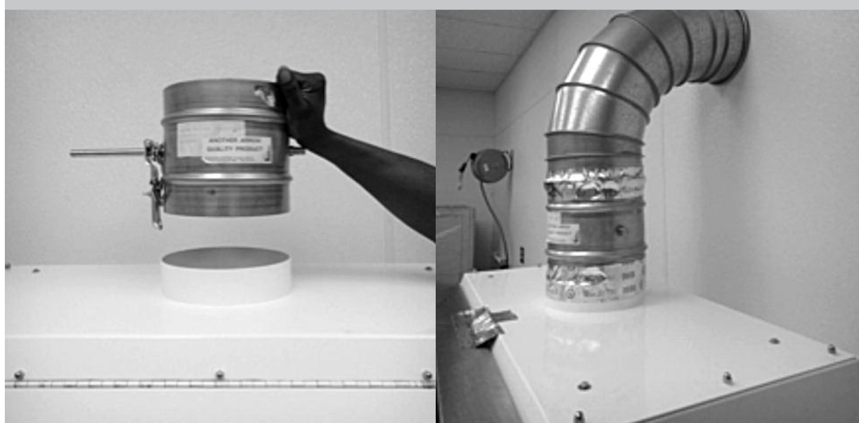
FIGURE 14. PLACING DAMPER AND ATTACHING DUCT
