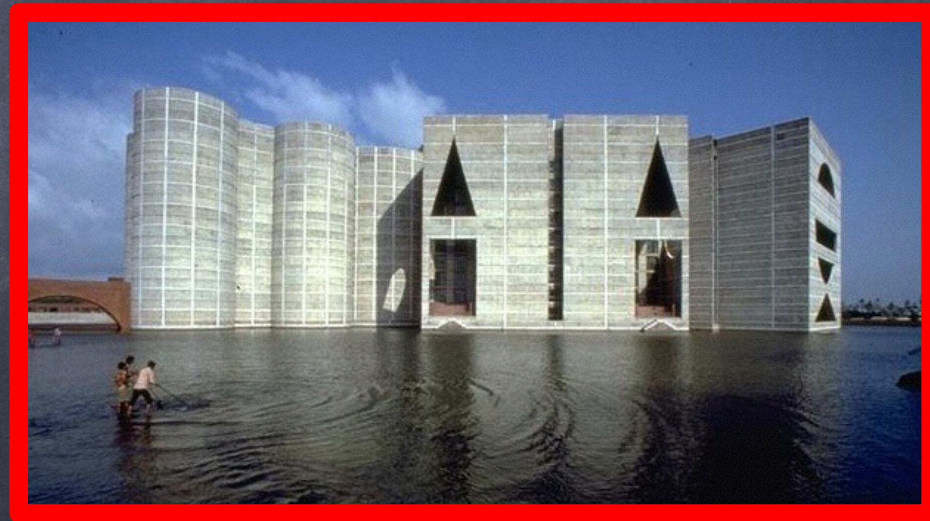
National Assembly Building, Dhaka
